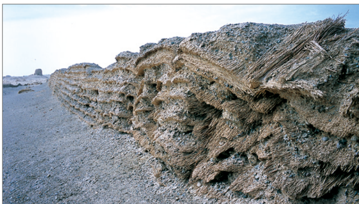
Figure 5: Western Han Great Wall located near Yumenguan, Gansu Province, China, made of reed stalks and earth. Photo by William Lindsay
