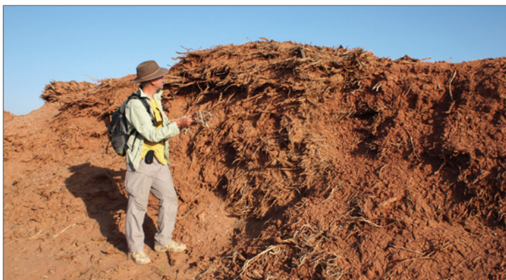
Figure 6: The author examines wooden material at a section of Genghis Khan Wall in Omnögovı consisting of saksaul branches and red earth. Photo by James Lindsay
