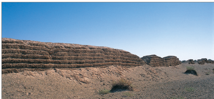
Figure 4: Western Han Wall located in Guazhou, Gansu Province, China, made of tamarisk branches and earth. Photo by William Lindsay
