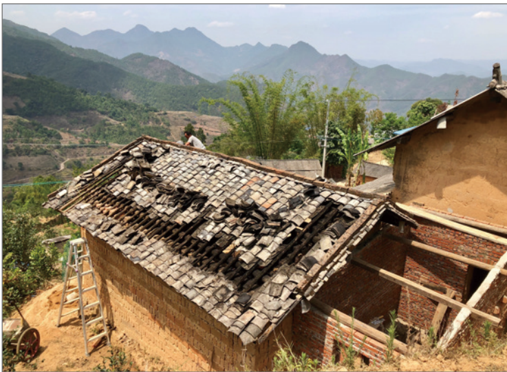
Figure 3: Renovating Landlord Li's Old House
